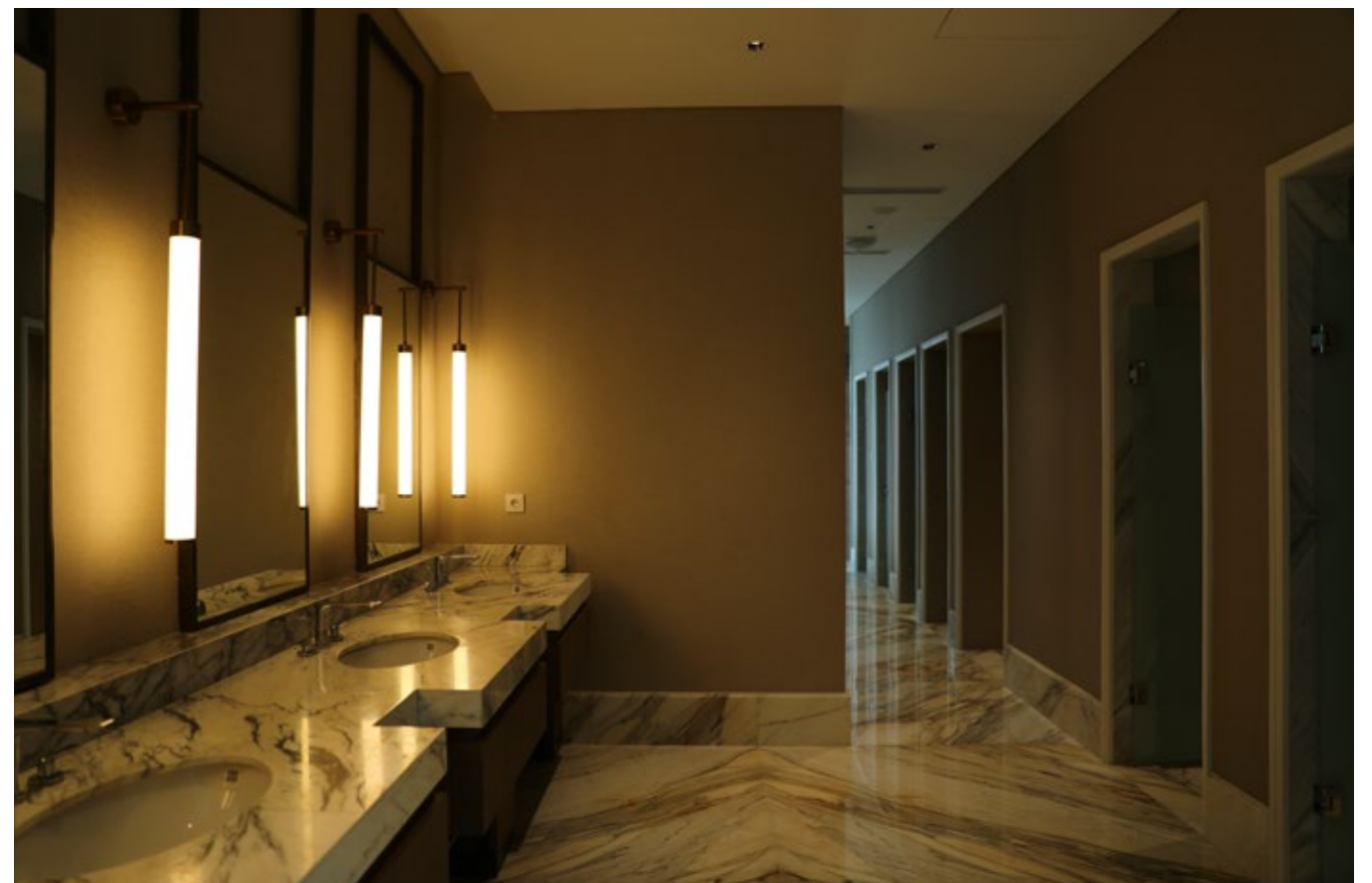
Changing Room. Steam and sauna will be finished in end of August. Finishing works is currently at 80%.
