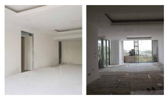
Marble installation for residence is starting. Homogeneous tile installation is in progress at basement 2 to 4 and level 3. Block wall partition installation reaches level 22
