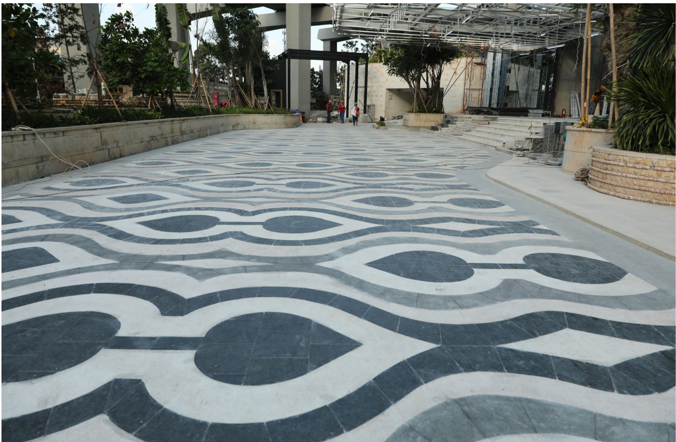
Lobby entrance driveway is 100% done.
