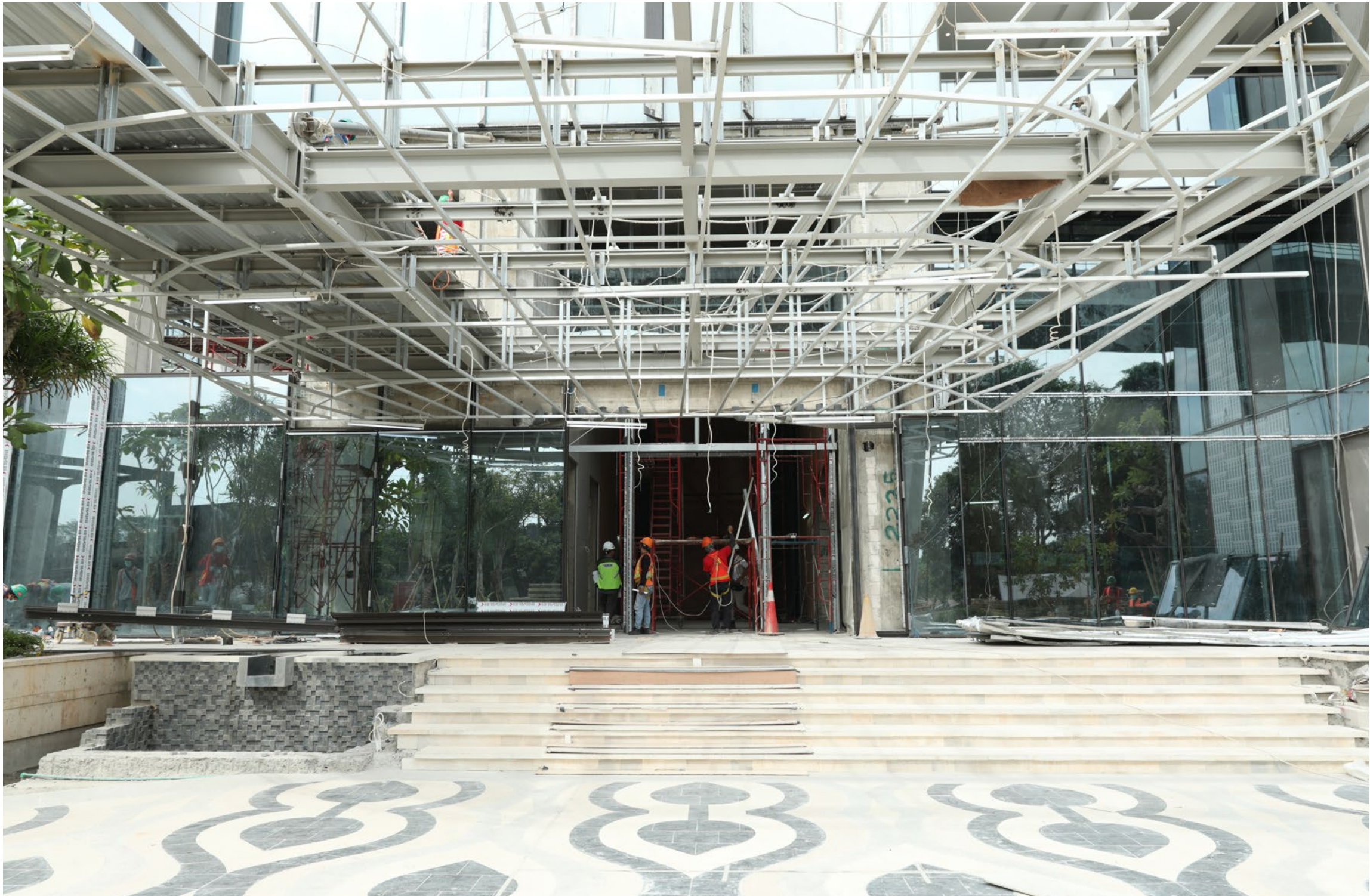
Lobby entrance with water features is 100% done.
